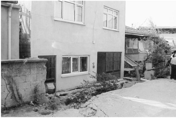
**Fig. 8.** Four-story building at Site F that underwent significant vertical and lateral displacement. Note gap between street and building that a felled tree was thrown in after the earthquake.
